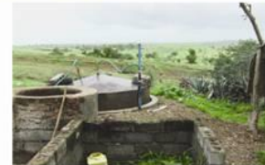
Bio Gas Plant
