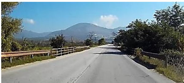
Dangerous guardrails (not a system)
