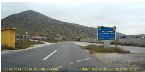
Missing access control (Route 6)
