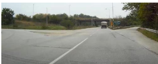
Missing channelisation in junction
