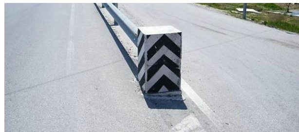
Dangerous “end treatment”- concrete block
