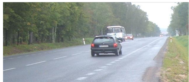
1+1 road with wide (asphalted) hard shoulders
