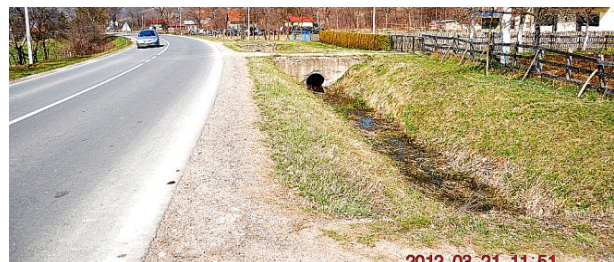
Unsafe drainage system, U-Type with headwall
