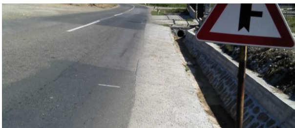
Unsafe drainage system, with headwall
