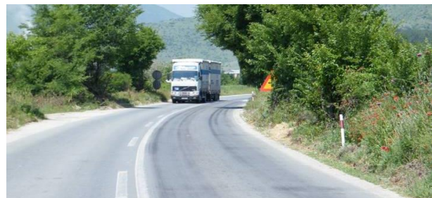
Insufficient site distance in curve
