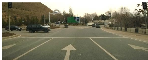
Missing channelisation in junction
