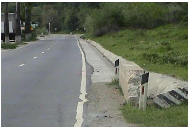
Unsafe headwall of a culvert
