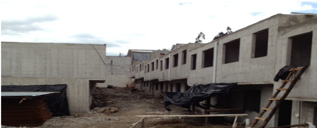
Low cost formal housing construction using poured in place concrete
