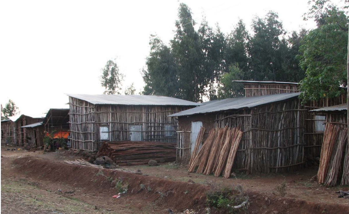
Picture 3 Squatter housing built with eucalyptus poles
