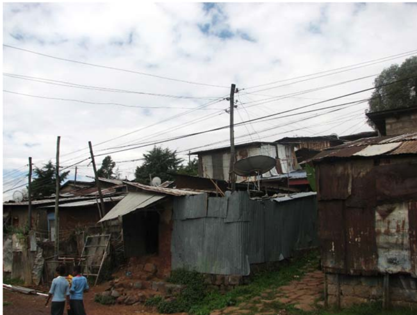
Picture 1 Informal power distribution
