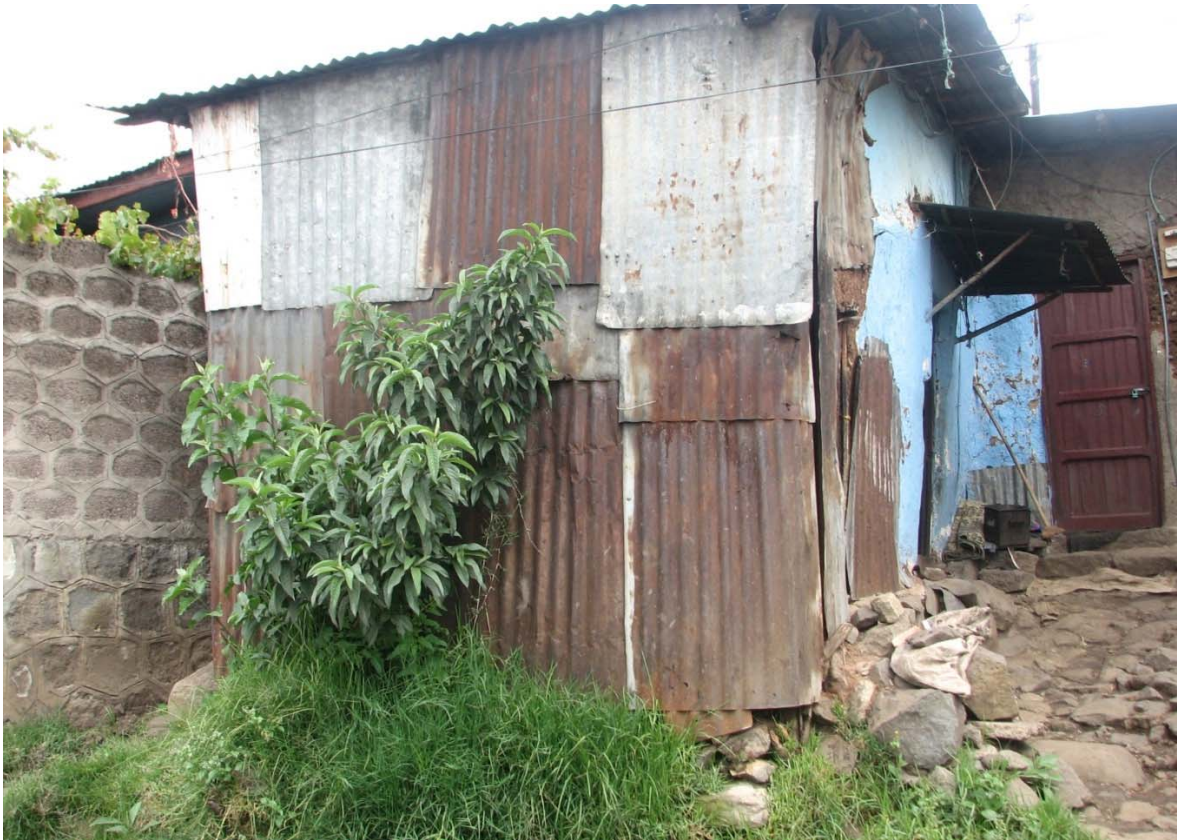
Picture 4 Squatter housing built with corrugated iron sheeting and poles
