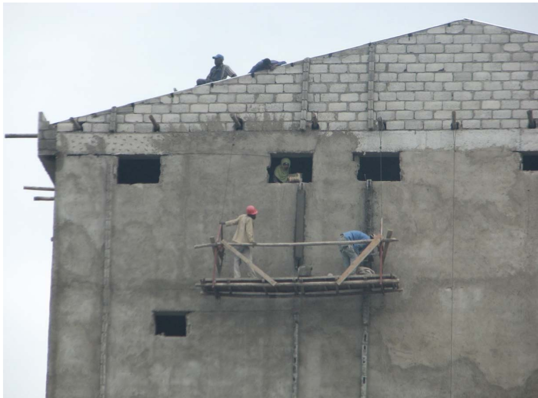
Picture 6 IHDP condominium construction
