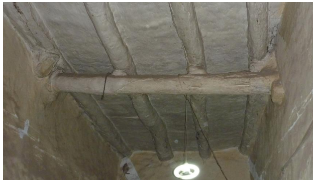
Interaction between floor beams and adobe wall
