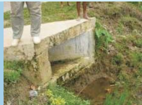
Scouring at the downstream end
