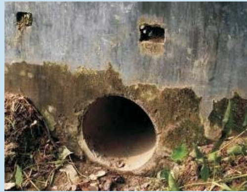
A single vent pipe culvert
