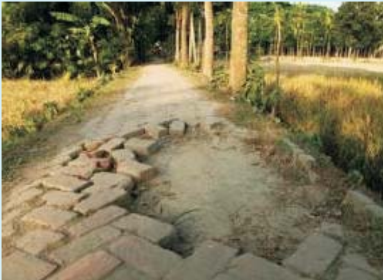
An edge that needs to be restored
