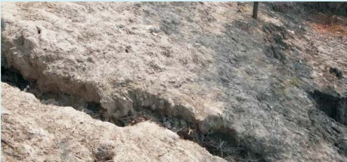
Rain cuts in an embankment
