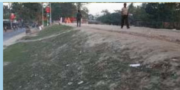
Well protected slope as turf has grown
