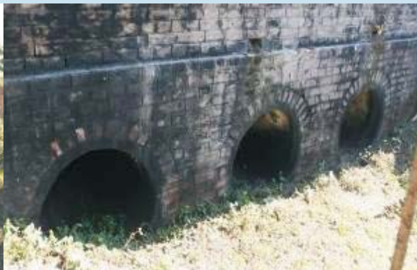
A three vent pipe culvert
