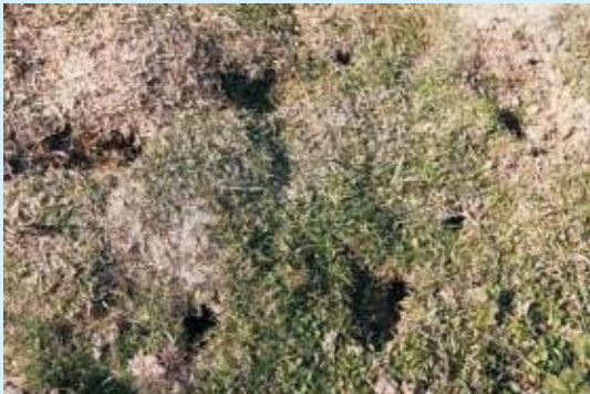
Rat holes on the slope of a road
