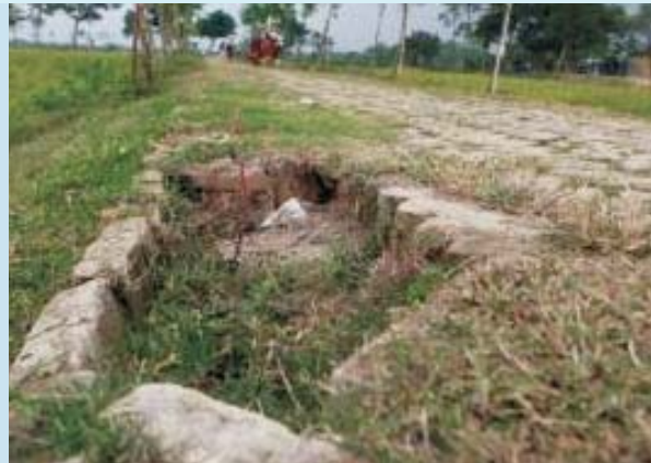
Bricks missing in a small area
