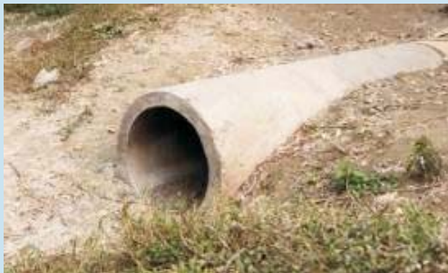
The end walls of pipes need to be covered
