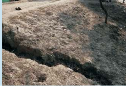
Rain cut causes damage to the road
