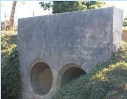
A two vent pipe culvert
