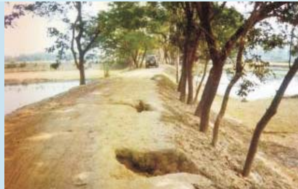
Rain cuts in an embankment
