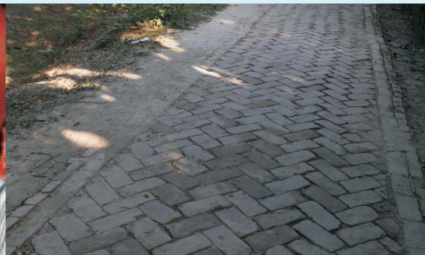
Bricks laid; the next step is the spreading of sand
