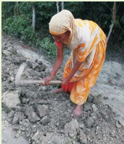
Break clods before compaction
