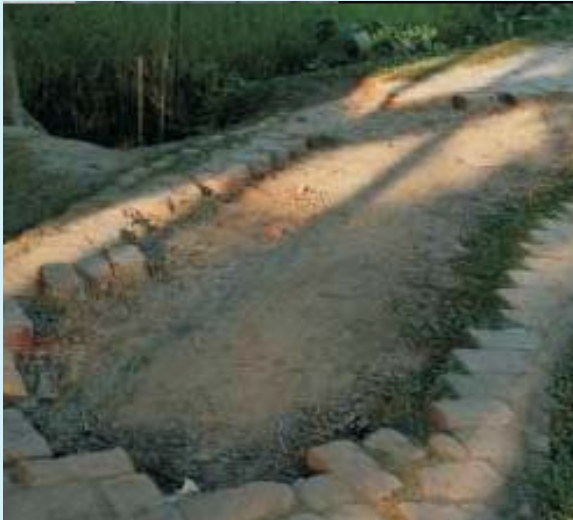
A BFS pavement damaged over a large area
