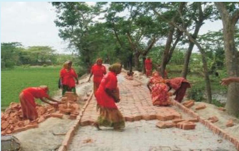
The top layer of bricks being placed over flat soling
