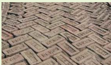
Use sand to fill in brick joints
