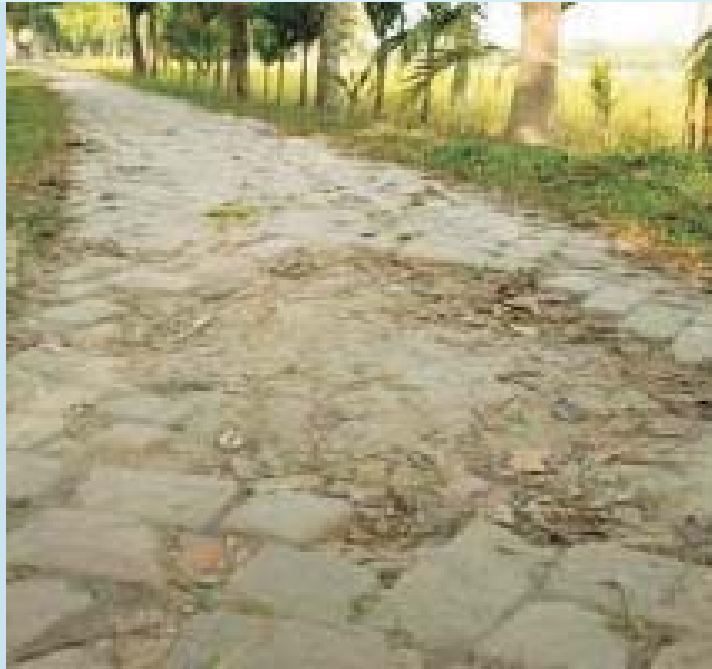
Damaged/missing bricks create potholes on the road surface.
