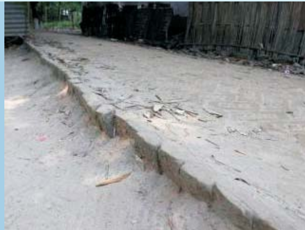
The brick-end edging has no support
