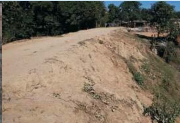
A damaged slope of a road
