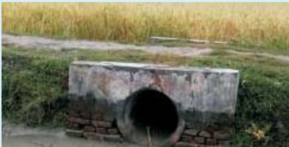
Pointing needed in the brick wall
