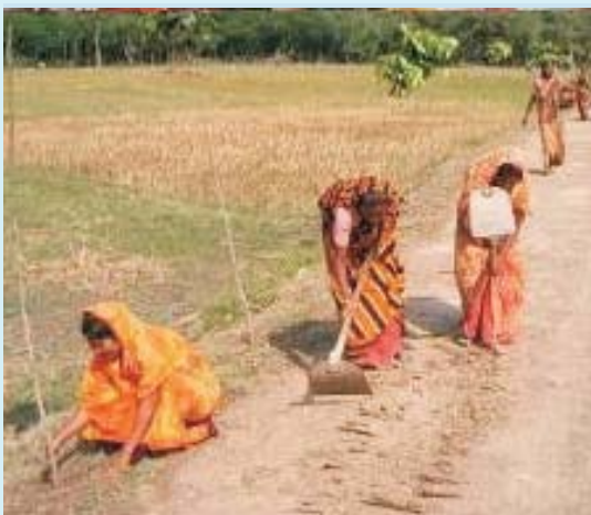
Raised shoulder being lowered
