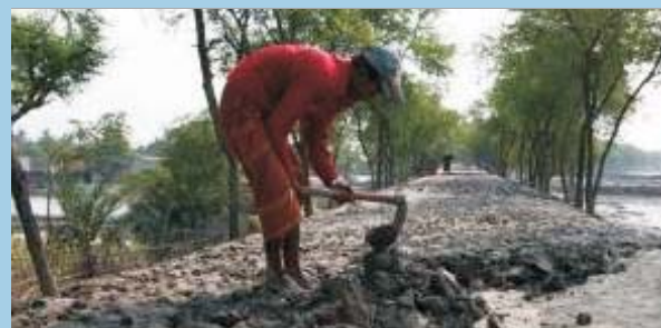
Layer placed ready for compacting
