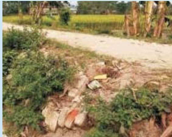
Edge and shoulder need to be restored
