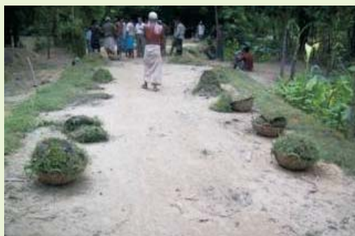
Use turf to protect soil from erosion
