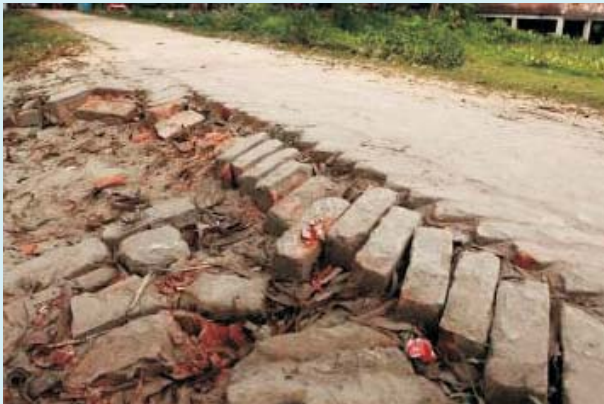
Main pavement under threat due to edge failure
