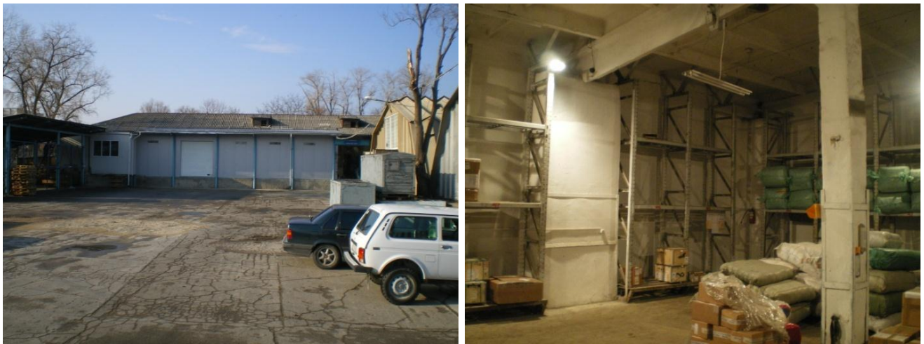
Figure 3.6. Air Cargo Warehouse at Chisinau International Airport
