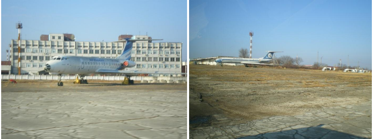
Figure 3.3. Apron of Air Moldova in Chisinau International Airport
