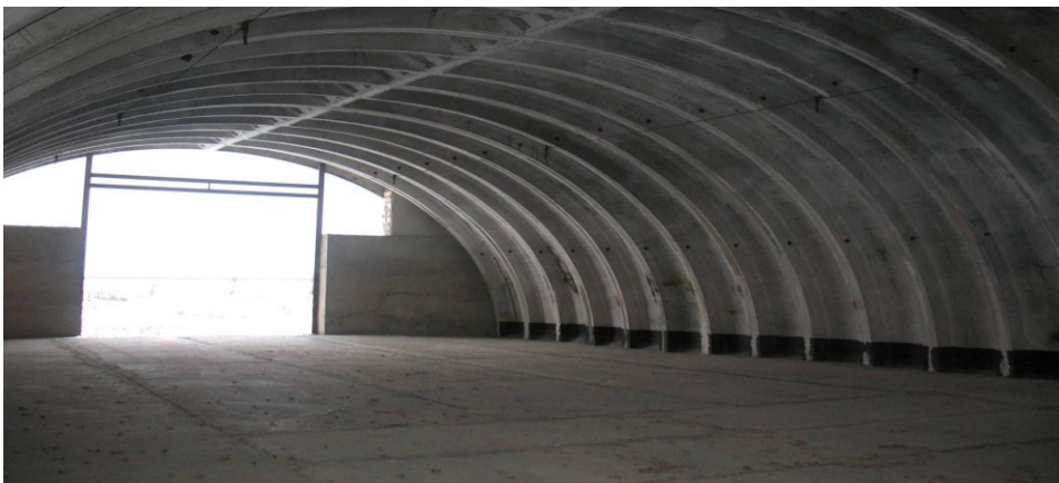
Figure 3.17. Hangar for Air Cargo Terminal
