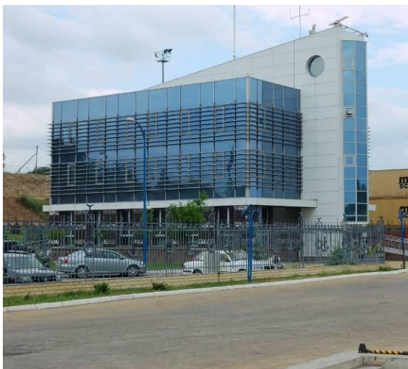
Figure 3.1. State Passenger Terminal Giurgiulesti
