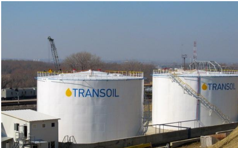
Figure 3.4. Vegetable Oil Terminal
