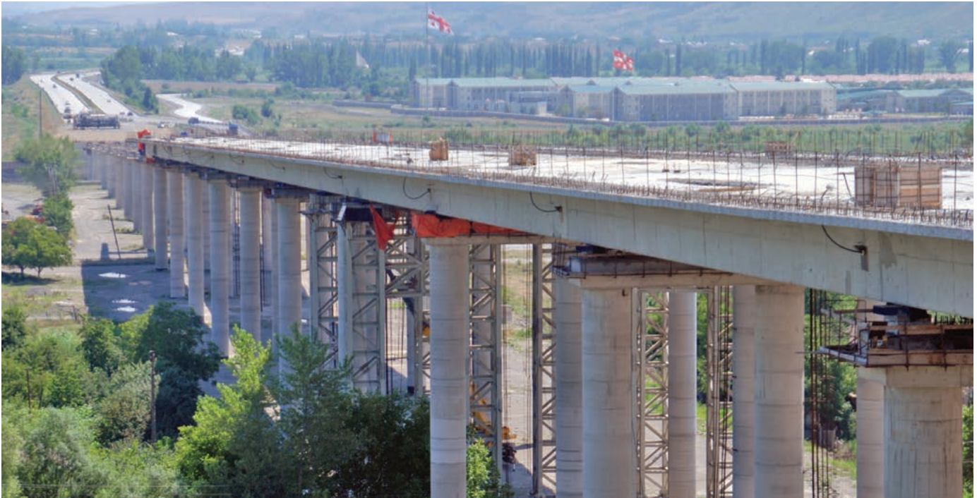
The Liakhvi bridge on the East-West Highway, built with the latest construction technology.
