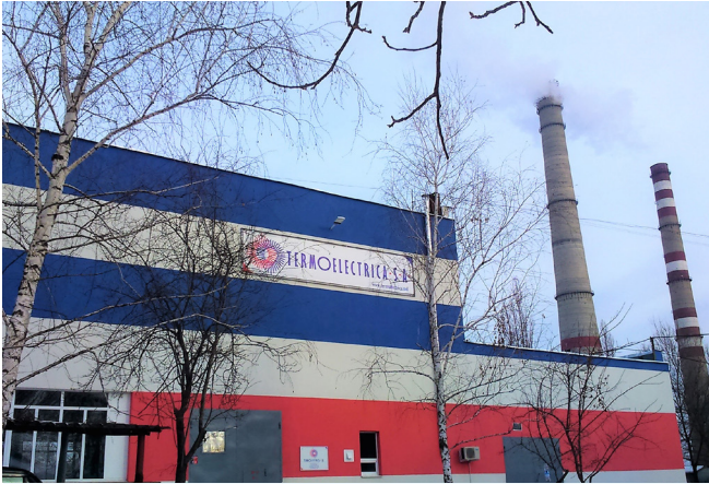
The new pumping station at Termoelectrica JSC helped to significant energy savings and CO2 emissions reduction.
