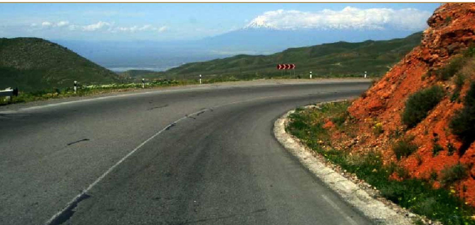
North–South Road Corridor, Ararat Region
