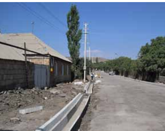
New drainage along the Zoravan–Aragiugh road
