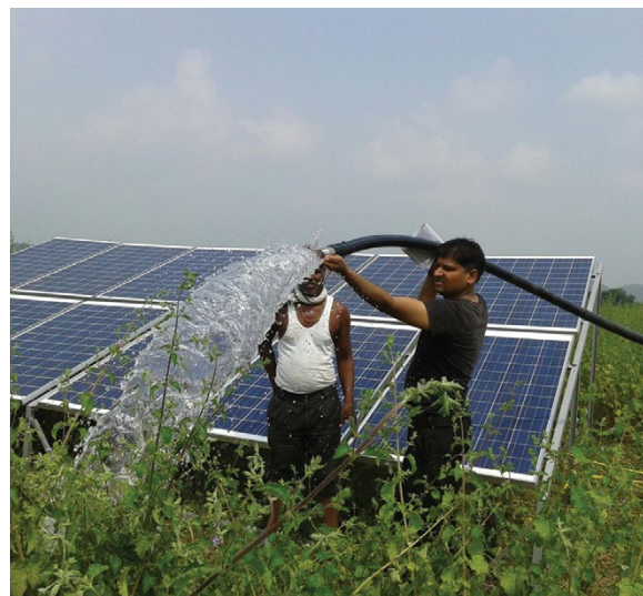
Solar water pump in India
