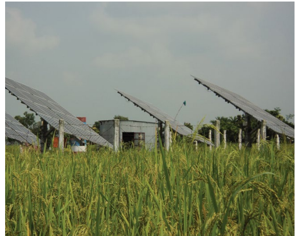
Grameen Shakti solar irrigation pump in Sapahar Noagoan in Bangladesh
