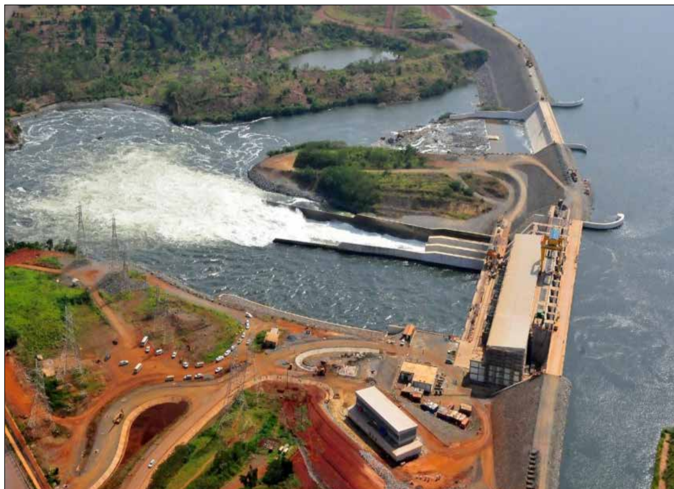
Figure 107: Aerial view of Bujagali hydropower plant
