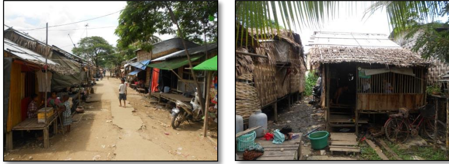
Figure 1: Limited access to the Government grid in YGN-3 28
