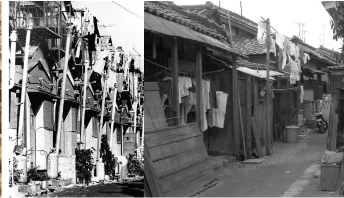
Inadequate and Dense Housing
