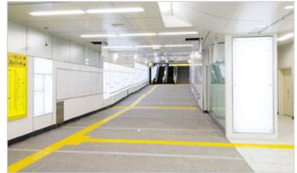
Bumpy warning tiles in bright yellow to guide blind passengers safely.
