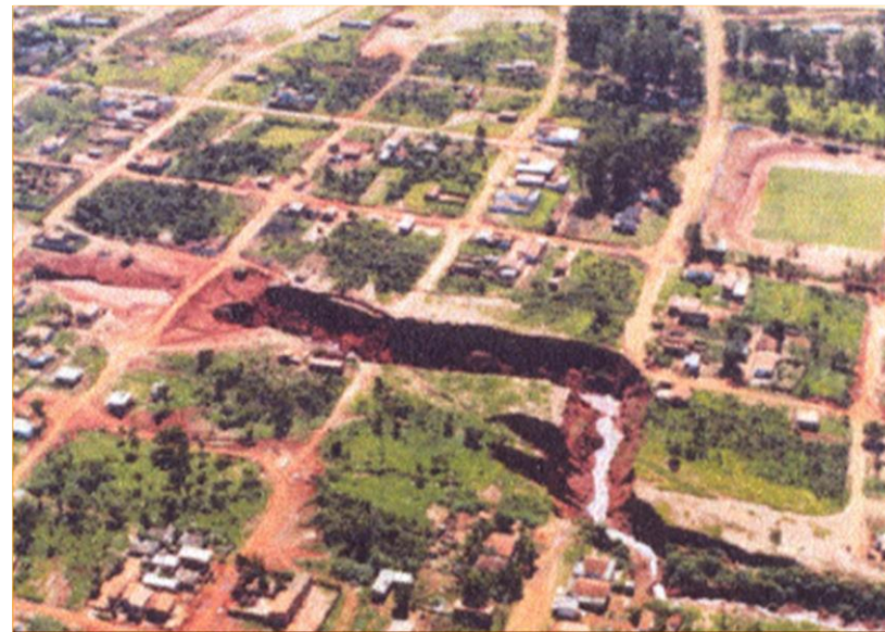
Degraded area by increase on flow velocity
