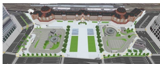
Figure 1: Image of Tokyo Station and completed multimodal transit terminal
