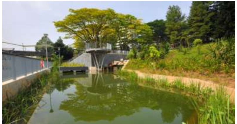
Sedimentation basin @ Sg Ulu Pandan
