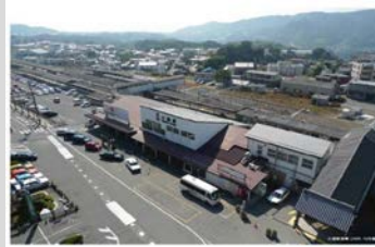
▲ Komoro Station front Closing of Nagano Shinkansen line drastically decreased the number of users.
