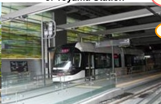
LRT space under the girder bridge of Toyama Station
