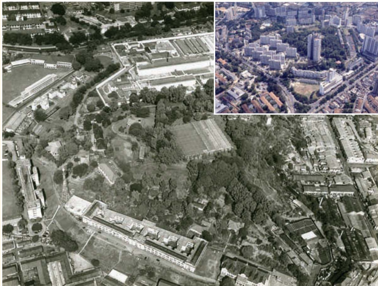
Photograph 10.2 Precinct S1 before redevelopment and after redevelopment
