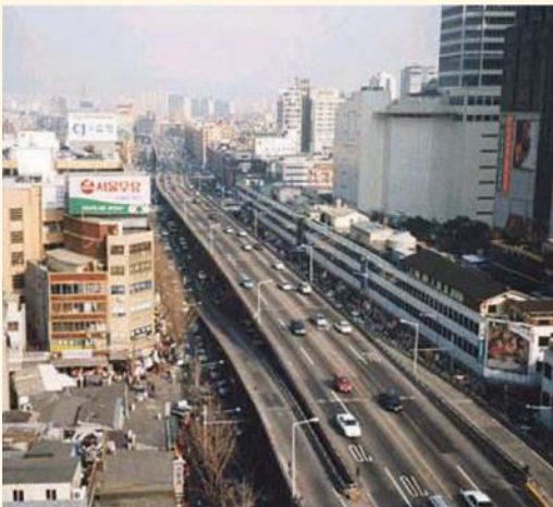
a. Before restoration
