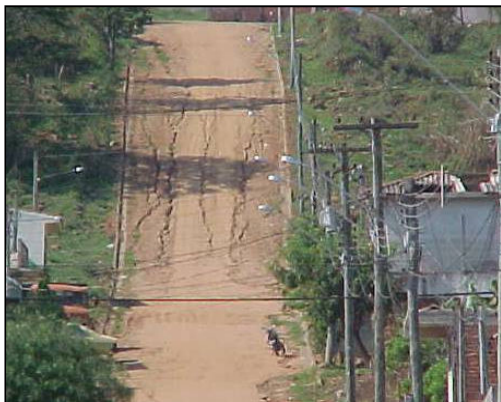
(b) Laminar erosion in street (source: eng. Luiz Orsini)
