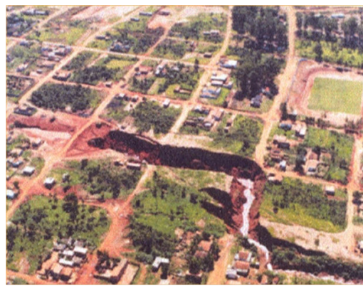
(b) erosion from velocity increase (source: prof. Nestor Campana)
