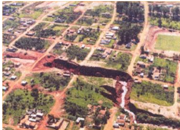
Degraded area by increase on flow velocity
