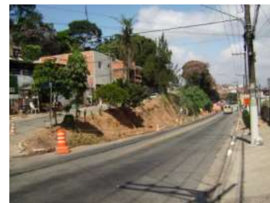
Av. Alda - before works
