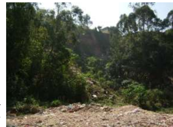
Pedra sobre Pedra slope – before works
