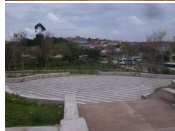
Linear Park – Reimberg Cocaia – after works
