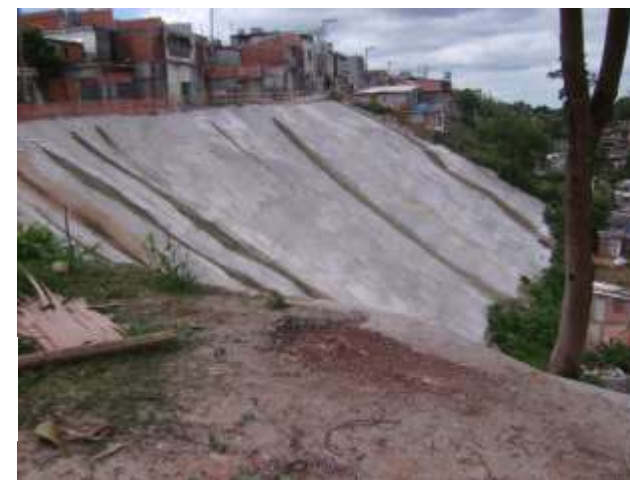
Rua Beira Rio – after works
