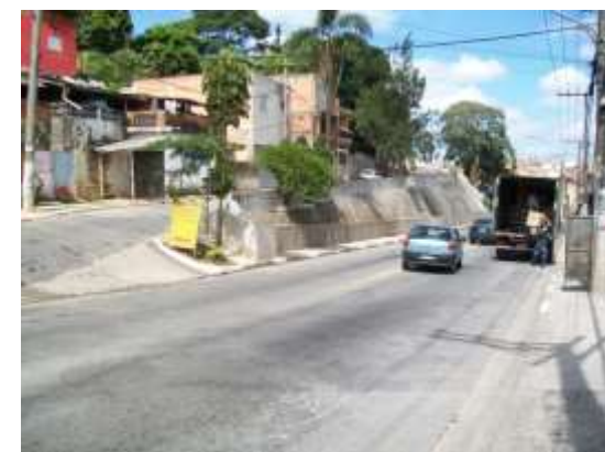
Av. Alda - after works
