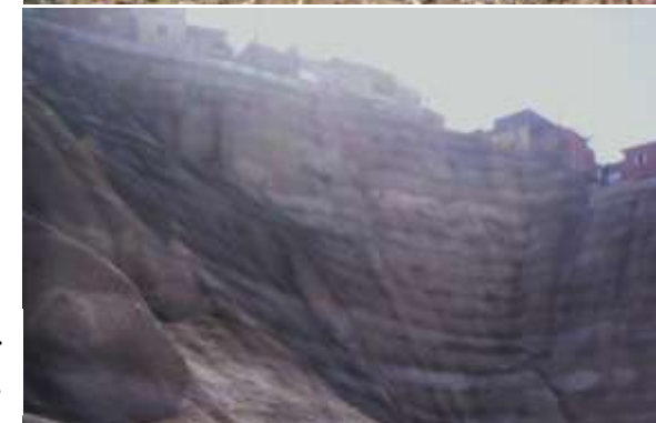
Pedra sobre Pedra slope – after works
