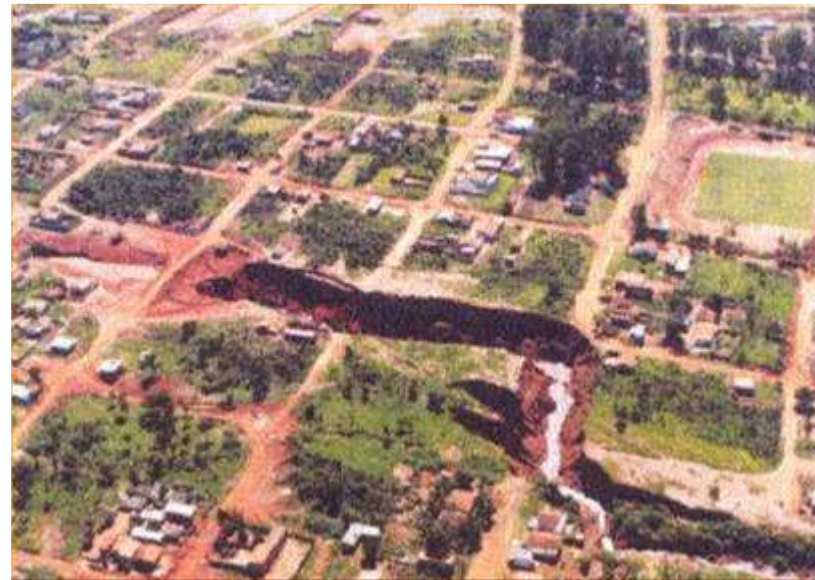
Degraded area by increase on flow velocity
