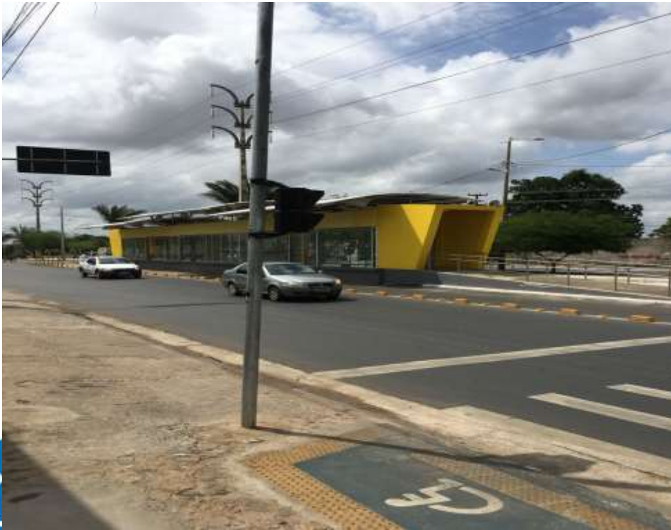
Exclusive bus corridor in Avenida Barão de Gurgueia
