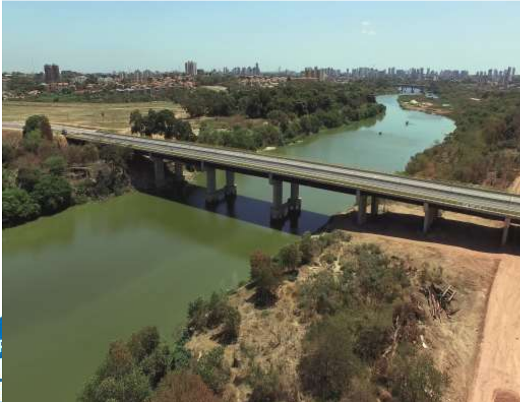
Implantation of a new bridge to connect the south and southeast of the city. Anselmo Dias Bridge
