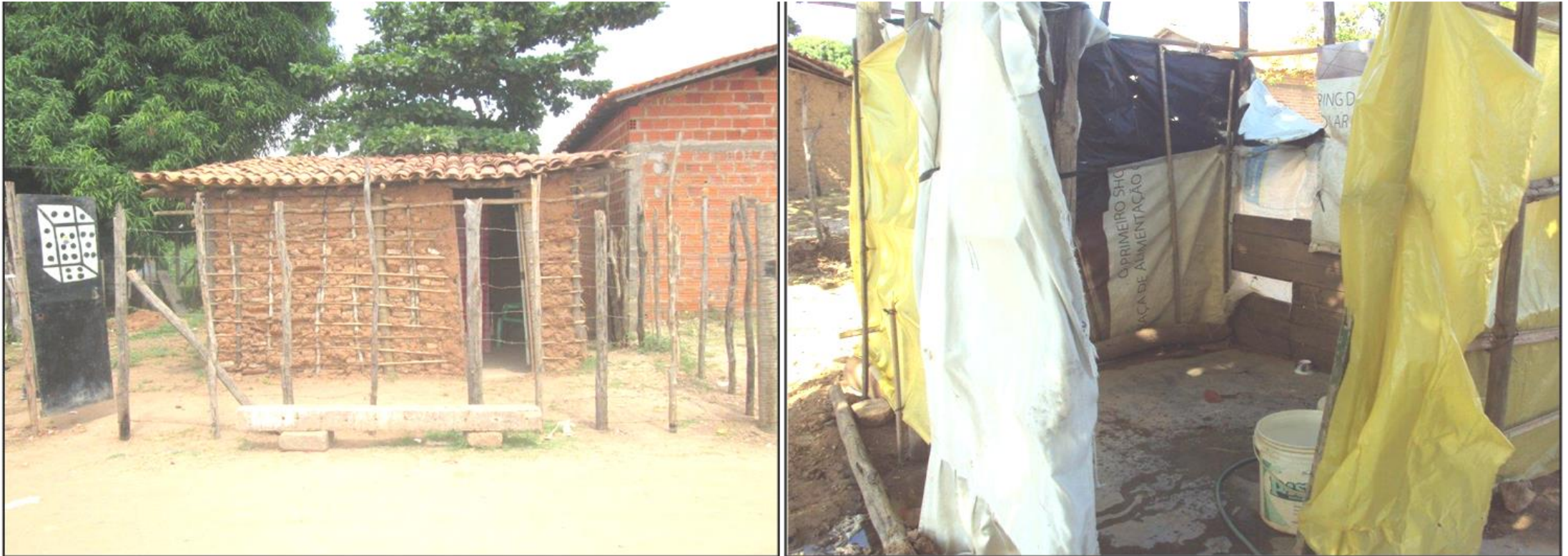
Figure 1. Example of a standard property estimated at 'Below Minimum' level. Left: façade of the building. Right: external improvised 'bathroom'.
