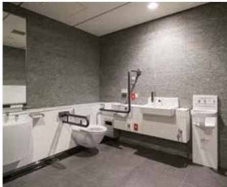
Installation of universal-access toilets
