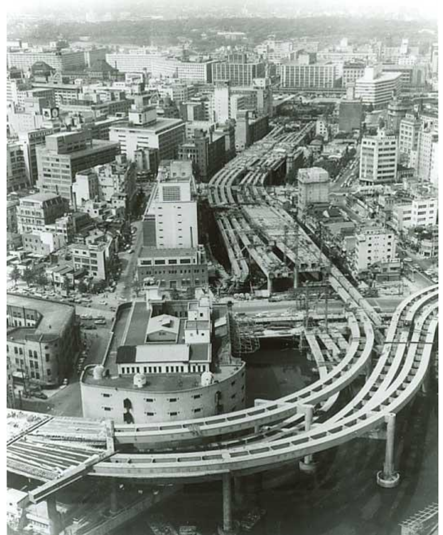
Tokyo Metropolitan Expressway
