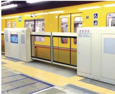
Installation of platform screen doors
