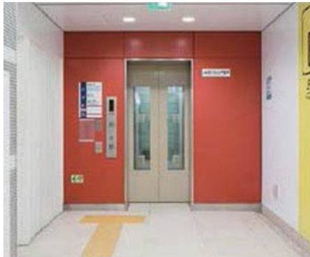
Installation of elevators, etc.
