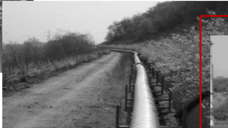
Construction of landfill gas transport pipes
