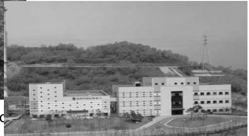
Heat production facility using landfill gas
