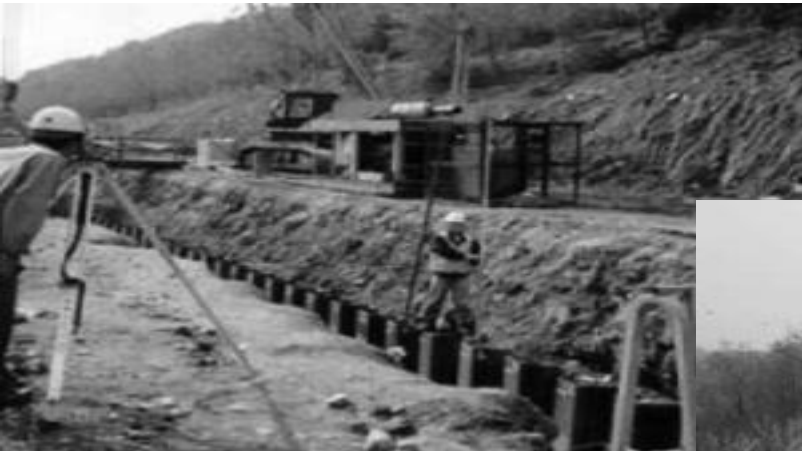
Installation of impermeable walls
