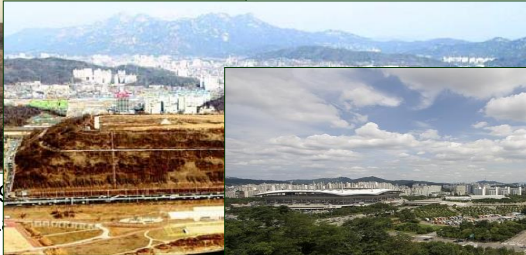
1996 ~ 2002 Stabilization and Construction
