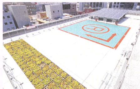
Rooftop landscaping, solar power system
