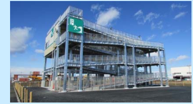
Tsunami evacuation tower at Nakano 5-chome
