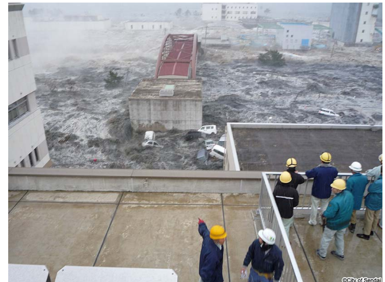
Sendai city's Minami-Gamo Wastewater Treatment Plant
