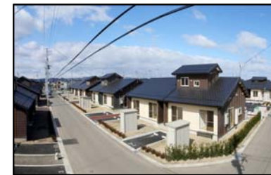
▲ Finished public housing
