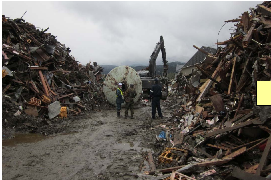
▲ Road-opening operation on a tsunami hit national road (taken on March 17, 2011)
