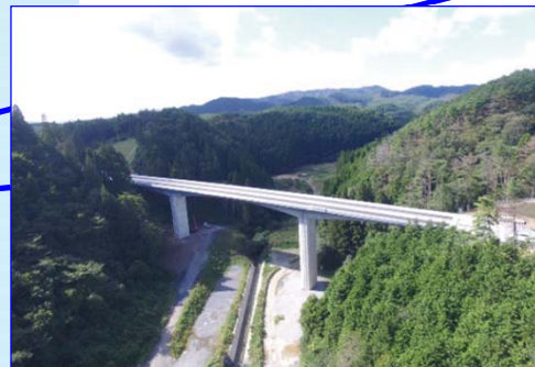
▲Completed Sanriku-engan road (opened to traffic on Dec. 9, 2017)
