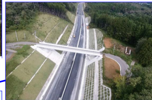
▲Restored Sanriku-engan road
