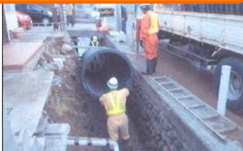
Restoration of damaged pipelines
