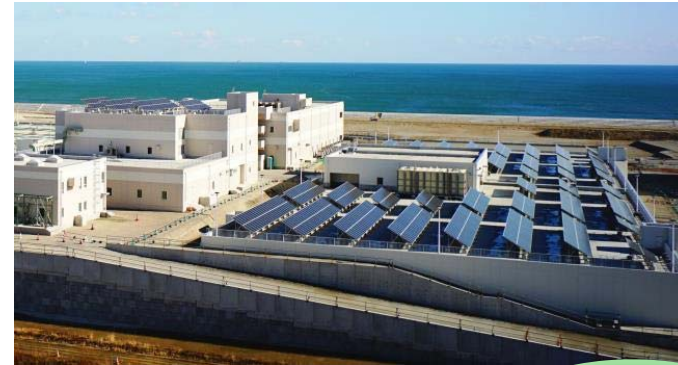
Tsunami-proof and eco-friendly facility (build-back)
