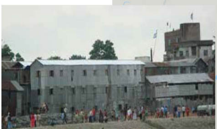
Timber and Bamboo Houses
