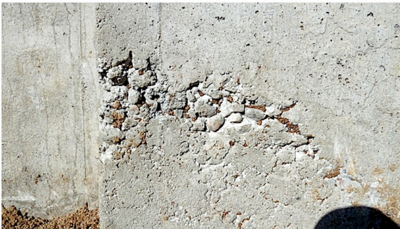
Poor concrete
