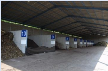
(2) Urban-type composting facilities
