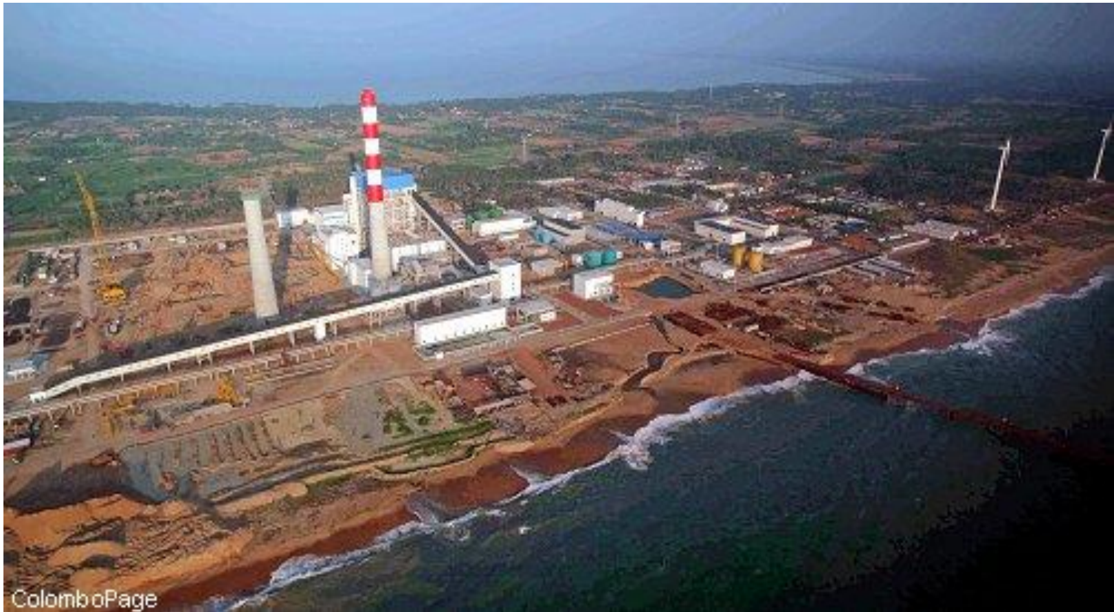
Puttalam Power Station in Sri Lanka
