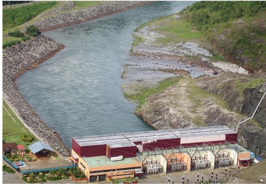
Sultan Mahmud Power Station, Malaysia
