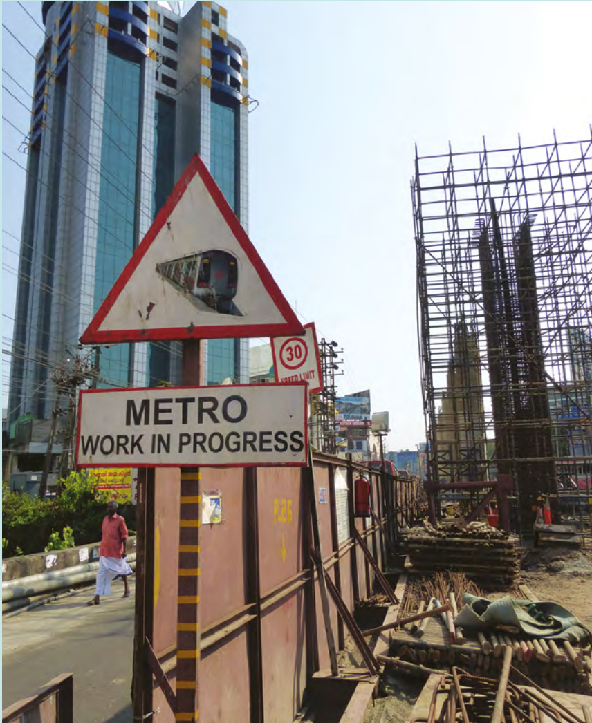
Figure 21 : Metro under construction in Kochi, Kerala State
