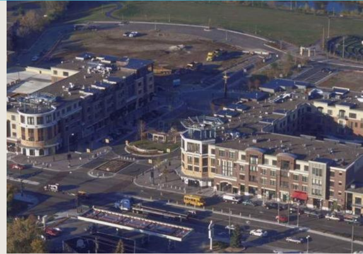
Corridor retrofit after
