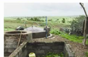
Bio Gas Plant
